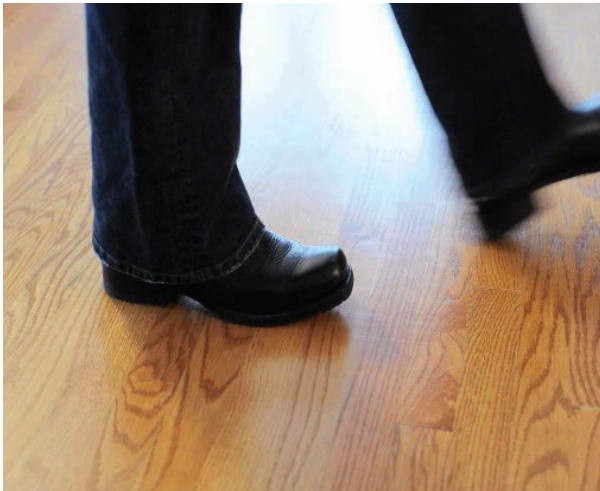
Figure 1. Sub-floor squeaks are a major percentage of customer complaints and callbacks in new residential construction.
